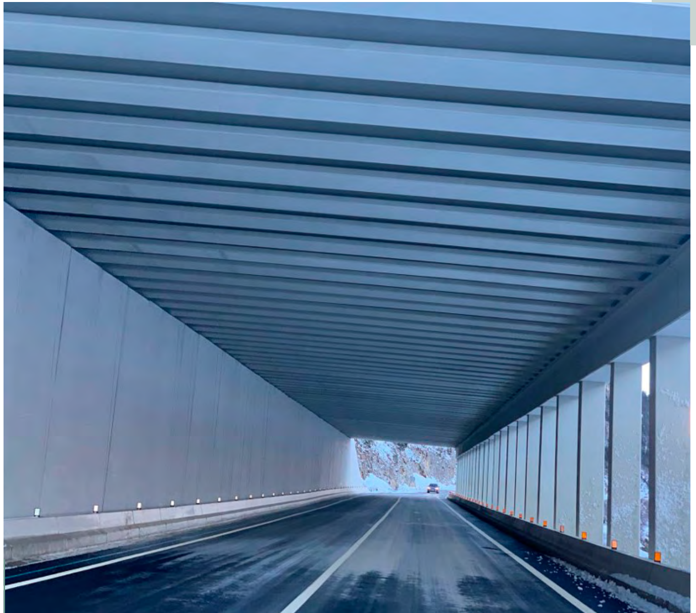
■ Avalanche protection gallery on C-28 road Baqueira (Lleida, Spain)
