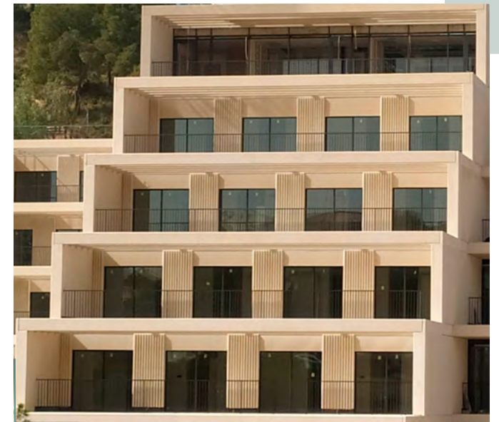
■ Residential with prefabricated structures in Malaga (Spain)
